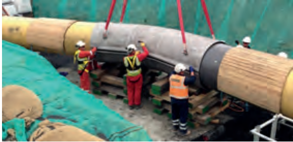
(a) Installation of fabricated shell at 30° bend
