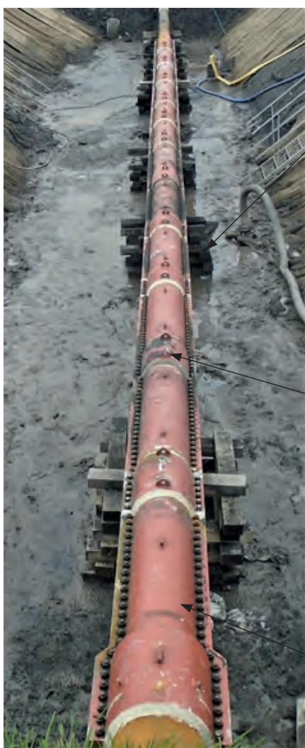
(a) Shells installed in excavation
