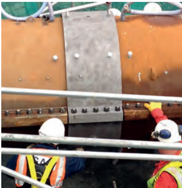
(c) Installation of continuity shell
