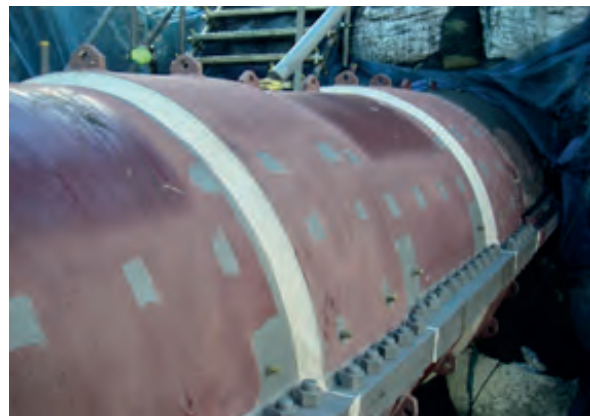
(e) Finish installation of continuity shells (note CP connection points)
