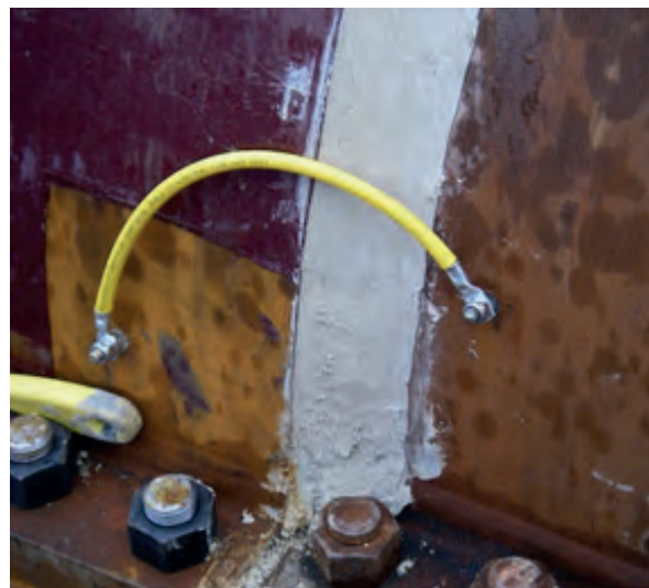
(f) Assuring electrical continuity for CP system
