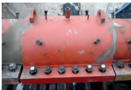
(c) Continuity shell (prior to sealing the ends and epoxy grout injection)
